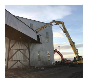
The two stacker/ unloaders boom and counter balance at super structure level was de-constructed by excavator and shear eliminating the need for operatives working at height. The super structure and base were then toppled by the excavator for further processing by machine and hot works operatives.
