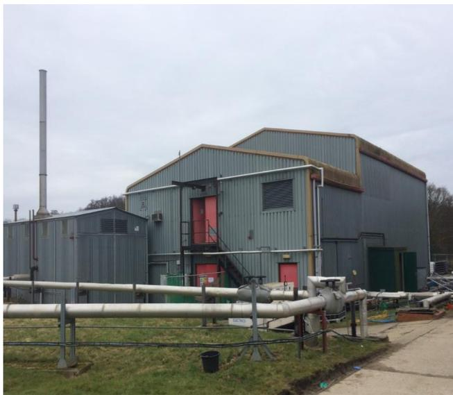
Demolition of the buildings were of a sensitive nature as for all the G/Waste generated from the works was stock piled and put through a shredder to go offsite as an energy from waste, and all scrap generated was processed onsite and went directly to smelter. All waste transfer notes corresponded with waste stream controlled by Ron Hull Demolition Ltd, all brick/concrete was transported to the laydown area for processing and crushed to a 6f2 material to be utilised onsite by the client.
