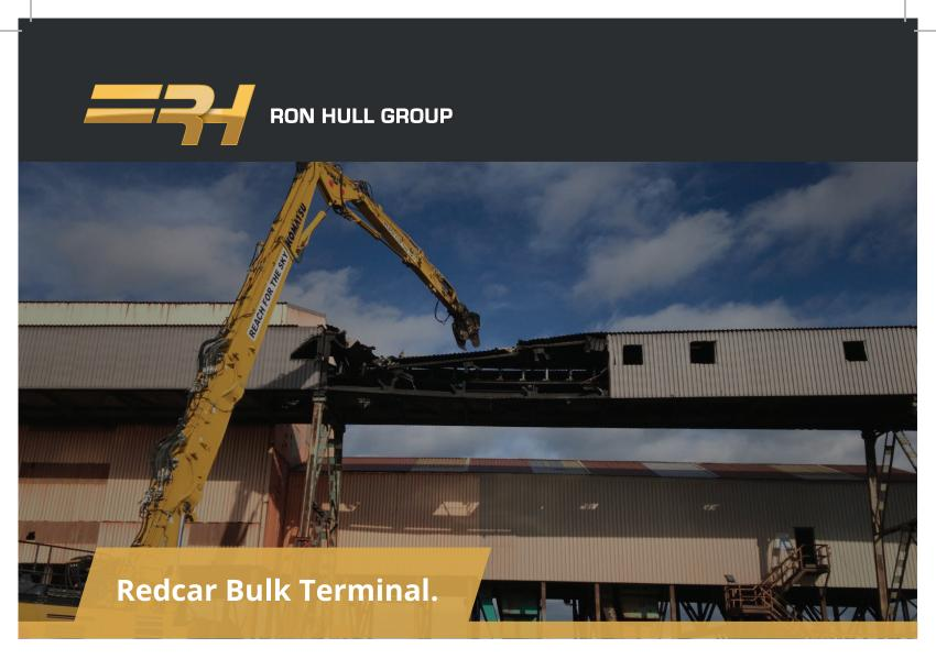
Ron Hull demolition limited was contracted by RBT to remove redundant conveyor systems at the above incorporating several transfer towers, drive towers, two 100m lighting towers and two stacker/unloaders weighing 350t each. The programme period for demolition and site clearance was 12 weeks, the contract was completed in 7 weeks.
